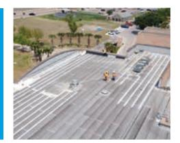
**Watertight**—EverSeal cures to a waterproof, tough, flexible sealant.
